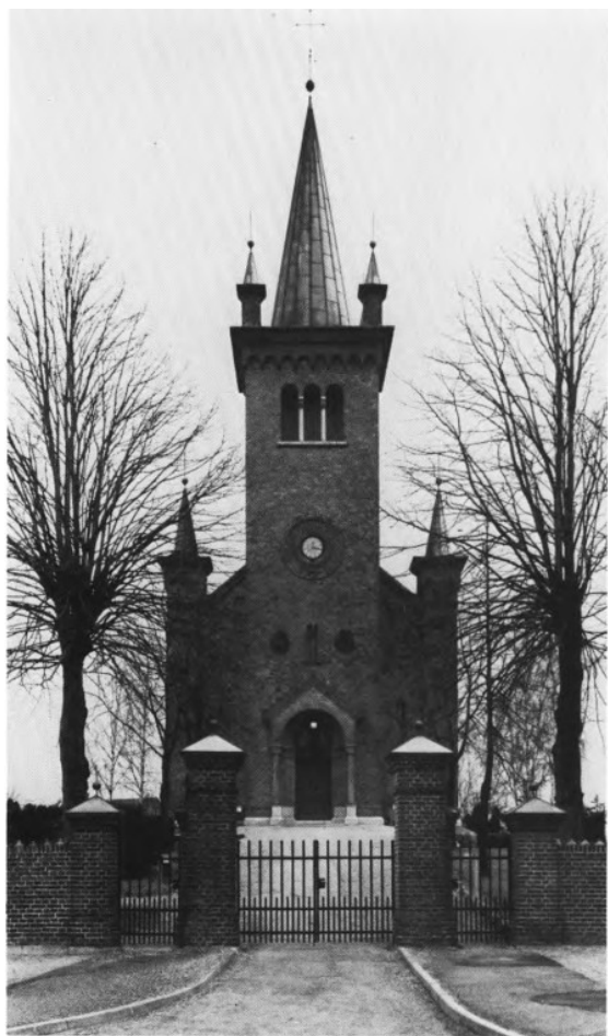
Fig. 2. Ydre, set fra vest. NE fot. 1981. — Exterior seen from the west.
